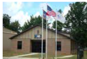
AKG Thermal Systems, Inc. Mebane, USA
