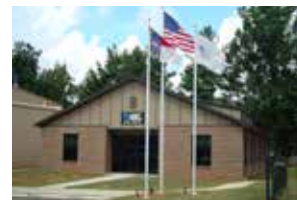
AKG Thermal Systems, Inc. Mebane, USA
