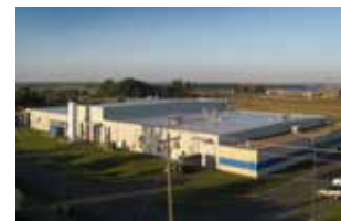
AKG North American Operations, Inc., Plant Mitchell, USA
