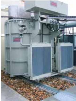
Stationary Oil Cooling for a power transforming plant, Bernard & Bonnefond
