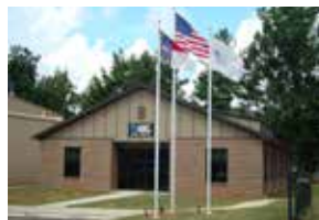
AKG Thermal Systems, Inc. Mebane, USA
